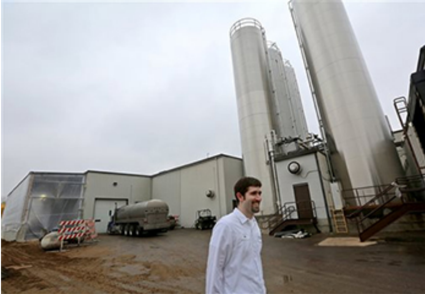
Plant manager Joe Steinocher makes his way past milk storage tanks near the Schreiber Foods receiving bay Thursday, March 27, 2014 in Richland Center, Wis. Schreiber Foods will begin construction of a distribution center this month in Richland Center to meet the growing demand for yogurt. The dairy giant has spent over $100 million in the last five years on its two Richland Center yogurt plants, which together employ about 400 people. (AP Photo/Wisconsin State Journal, John Hart)
