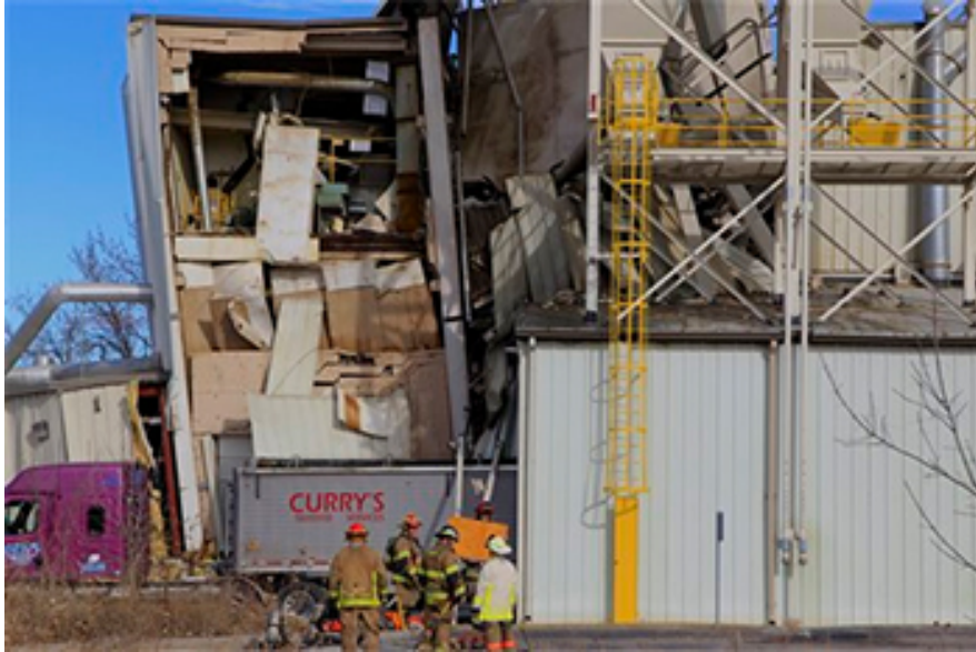
Firefighters stage outside the International Nutrition plant in Omaha, Neb., Monday, where a fire and explosion took place Monday, Jan. 20, 2014. Two people were killed and 10 others were seriously injured, authorities said. (AP Photo/Nati Harnik)
