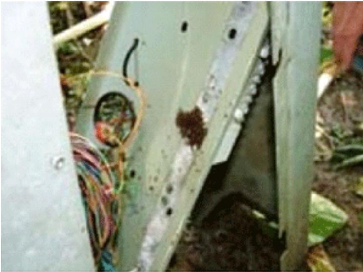
Large numbers of tawny crazy ants have accumulated in electrical equipment, causing short circuits and clogging switching mechanisms, resulting in equipment failure.
